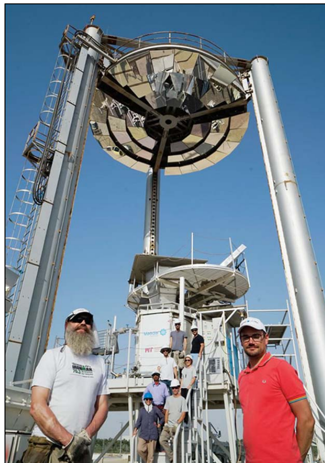
In the hot desert of the United Arab Emirates, Profs. Alexander Slocum (left) and Nicolas Calvet flank other research colleagues at their prototype of a Solar Beam Down Tower, which uses the sun to melt a stockpile of salt as a way to store clean energy.
