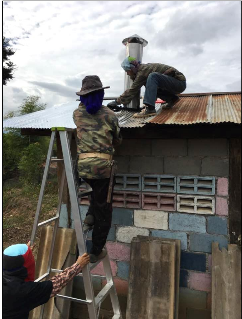
Above: Chimneying a stove through the aluminum roof of a cement-block house in a village in Chiang Mai Province, rural northwestern Thailand.
